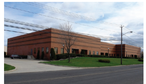
8500 REMINGTON AVENUE 12,800 SF | Pennsauken | LEASED!
